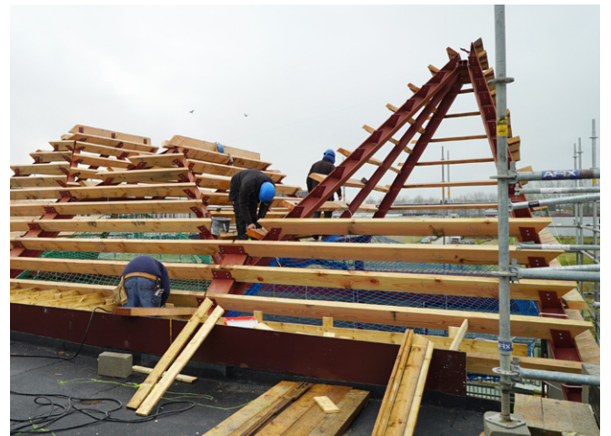
Diamond roof steel and wood framing under construction
